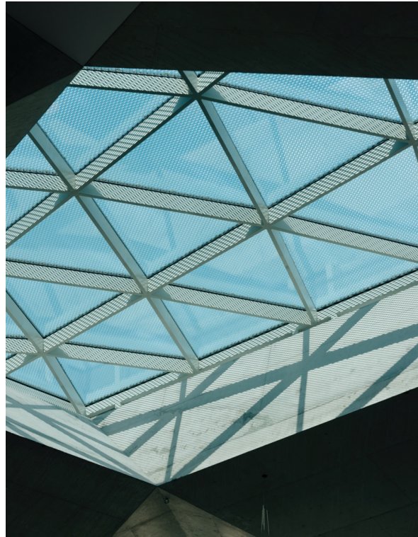
Okalux_Deichman-Bibliothek_@Einar_Aslaksen_03 The OKATECH wire mesh insert in the cavity between the panes sets visual accents and complies with high sun and glare protection requirements.
